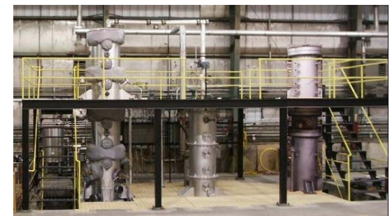
Coal Gasifier @ U of Utah
