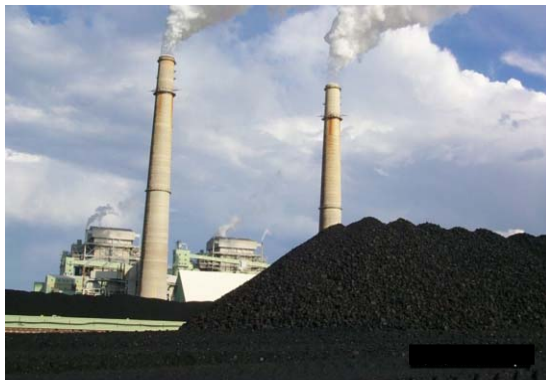
Coal-fired Utility Boiler
